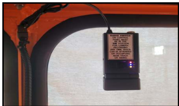
Outward Facing Camera Installed
